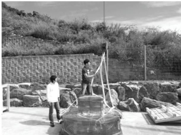
E. Lower the base frame onto the floor and remove the lifting assembly.
