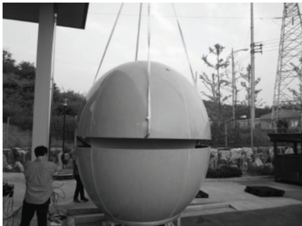
E. Once placed onto the lower half fasten with the supplied nuts and bolts. Then clean off any excess silicon.
