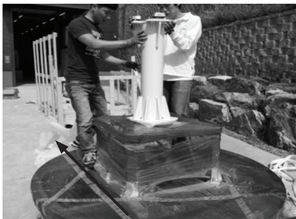
With the direction of the bow in mind, place the post on the top of the base frame.
