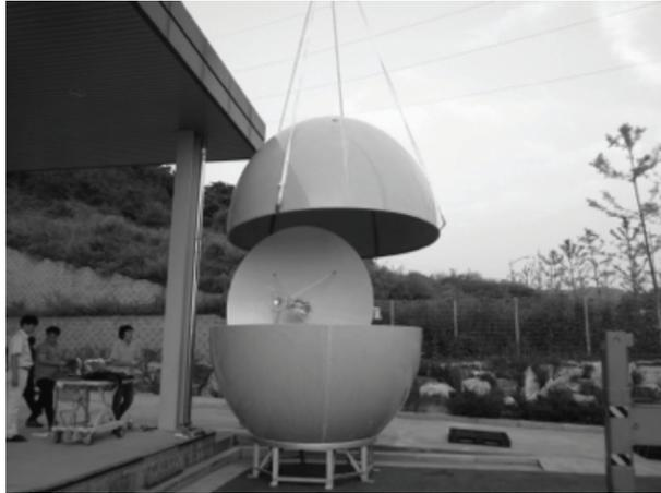
D. Apply silicon to the top lip of the lower section of the radome then slowly place the upper radome on to the lower radome half. Slowly place the upper radome on top of the lower radome assembly.
