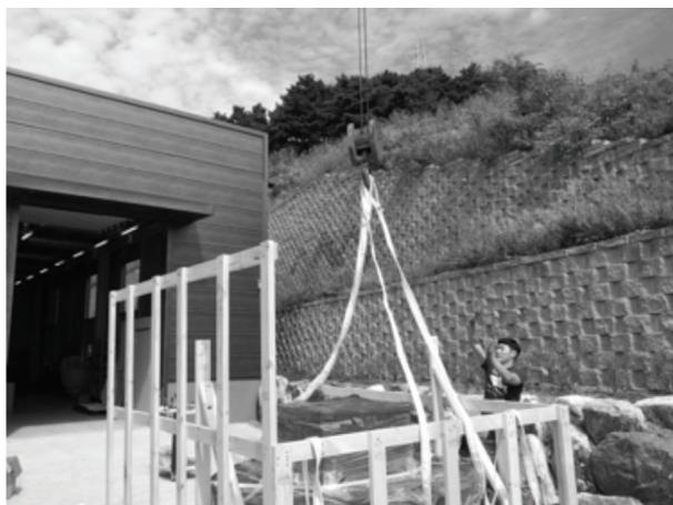
C. Make sure that the center of Base Frame is located right below of hook of Crane to create a good center of gravity and perform safe removal of base frame.
