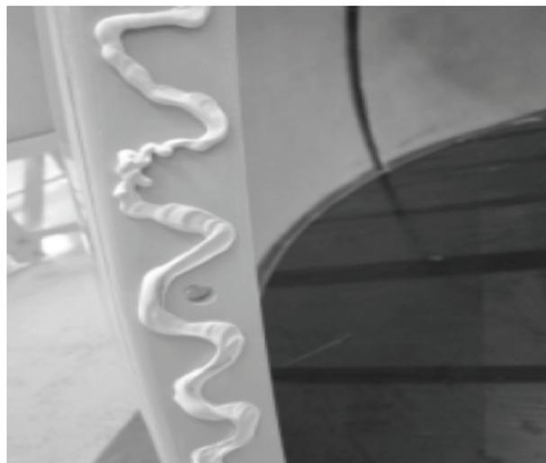
C. Apply silicon (Sikaflex-291) to side of radome panels before applying bolts.
