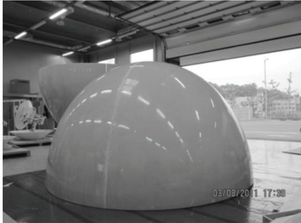
D. After the attachment of the cap, the last panel of the radome should be installed to finish the assembly. The final section is completed with a person inside the radome so a provision needs to be made so they can be released by lifting the completed dome. At this point all bolts should be tightened. Any excess silicon should be removed to give a clean finish.
