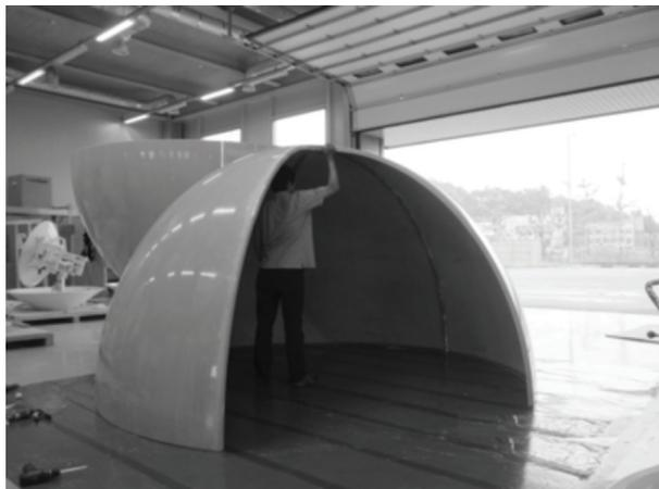
C. Fix the cap in place with a layer of silicon and loosely fasten the M6 bolts but do not tighten them at this time.
