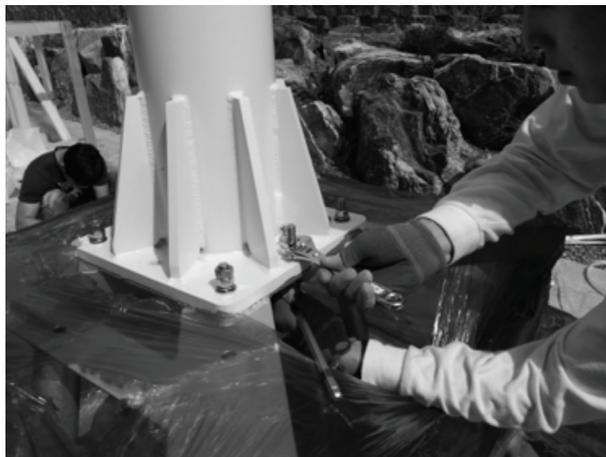
D. Secure the lower pedestal to the base frame with the 8 M12 x 60 bolts supplied. Lock the bolts by installing double nuts onto the bolts. Make sure to apply Loctite 262 to the bolts to securely tighten the assembly.
