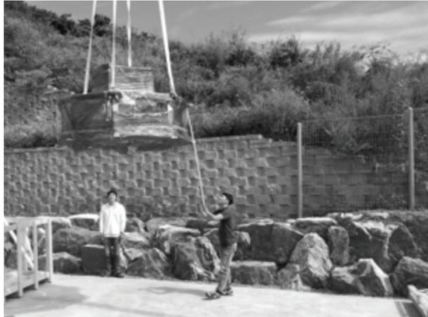
D. Very slowly lift up the base frame and watch as the base frame lifts up to prevent big interference with wooden crate.
