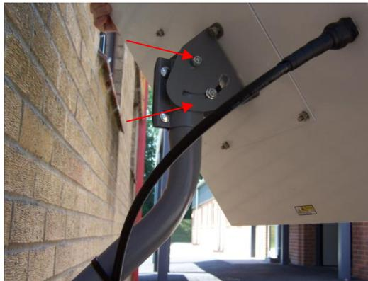
Figure 4-15 - Adjusting elevation
