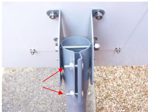
Figure 4-16 - Adjusting azimuth
